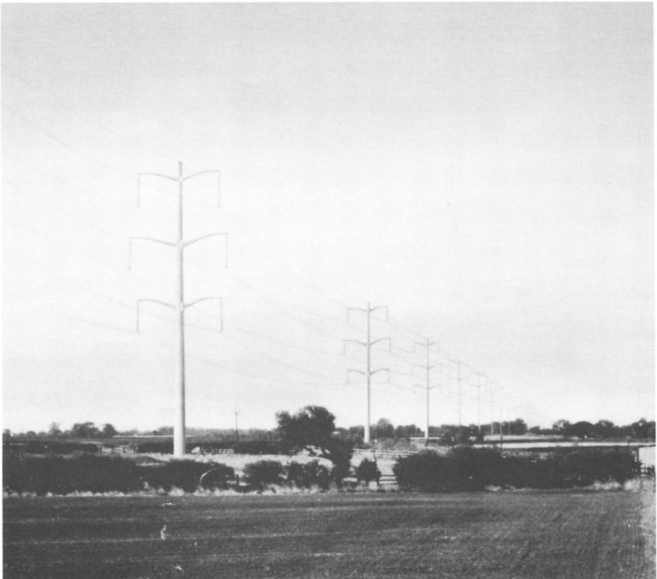
Figure 12 Generic tower types, folded plate pole (gull wing arms)
